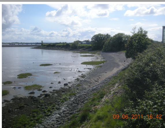
Photo 7: View from the top of the embankment (above the pumping station in Photo 2) looking west. Airport infrastructure assets located immediately behind the embankment.
