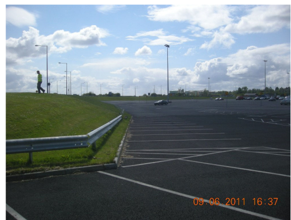
Photo 4: Airport car park showing significant difference in elevation between car park and embankment crest (approximately 2.0m).
