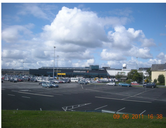
Photo 3: Airport car park and other infrastructure located directly behind the Shannon Embankments at a lower level than the estuary inter-tidal zone. Photo taken from top of embankment.
