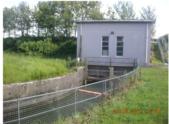
Photo 2: Pumping Station located at the end of a major back drain close to Shannon Airport.
