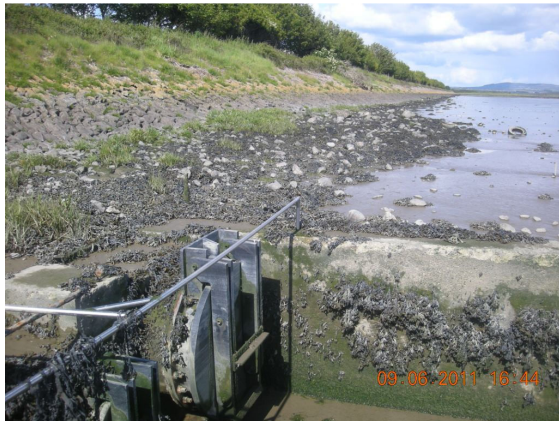
Photo 1: Embankment and back drain outfalls close to Shannon Airport.
