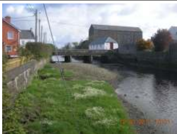
Photo 1: Ballylongford Bridge from the south d/s
