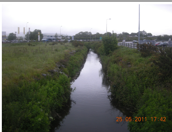
Photo 3: Looking u/s on the river diversion east of Tralee
